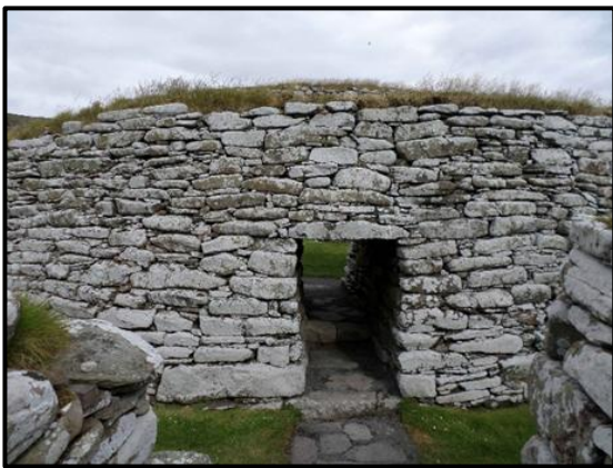
The access tunnel
