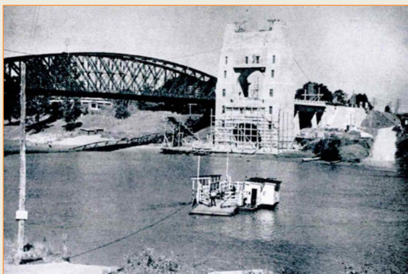
The Walter Taylor bridge under construction with the Indooroopilly Ferry crossing the river.
