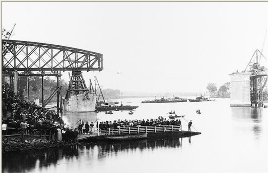
After a section of the Albert Bridge at Indooroopilly was washed away in the 1893 flood, repairing the railway link between Brisbane and Ipswich was a priority for the government. Crowds witness the launching of a new bridge span along the Brisbane River 1895.
