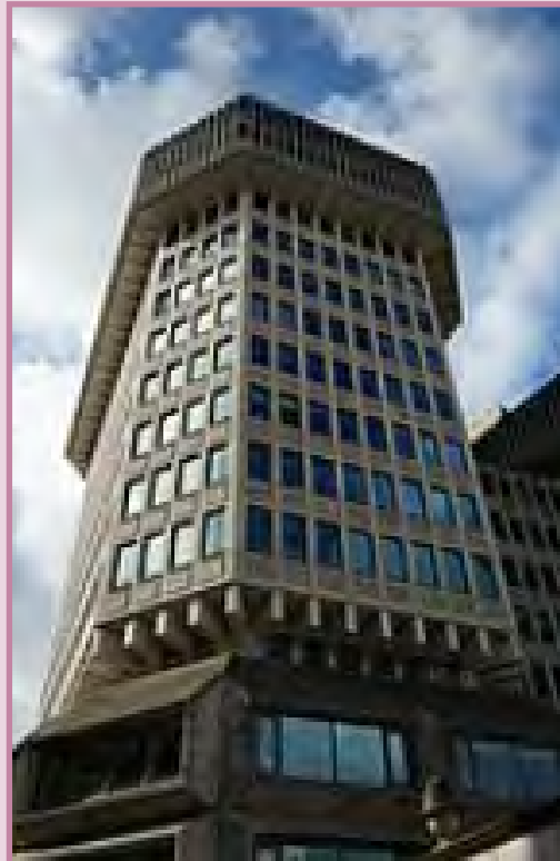
Ministry of Justice Building
