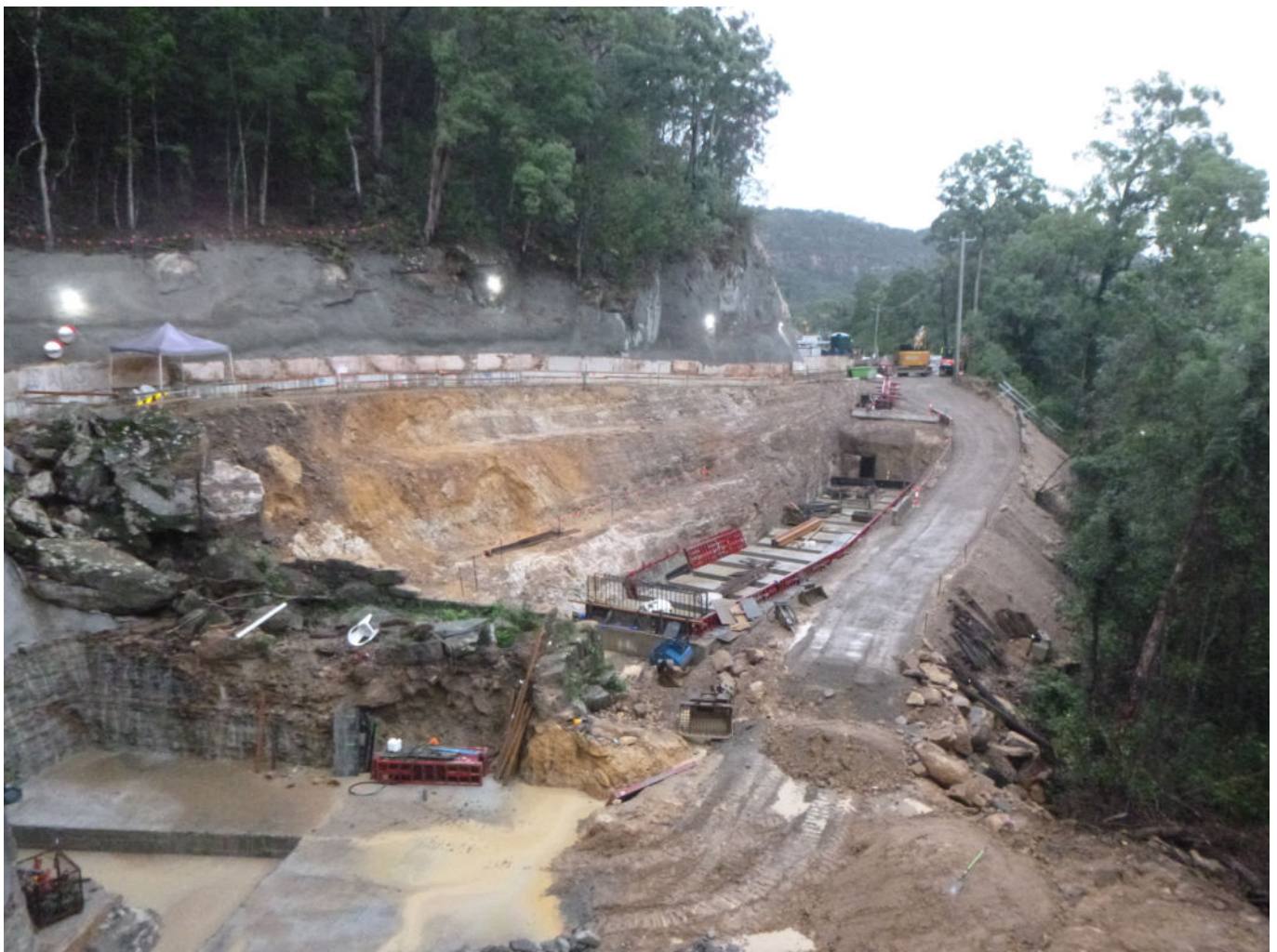
Photo taken from same position as photo taken on 20 April showing the progression in the works despite the wet weather. Concrete base poured on Devines Hill side of bridge base.
