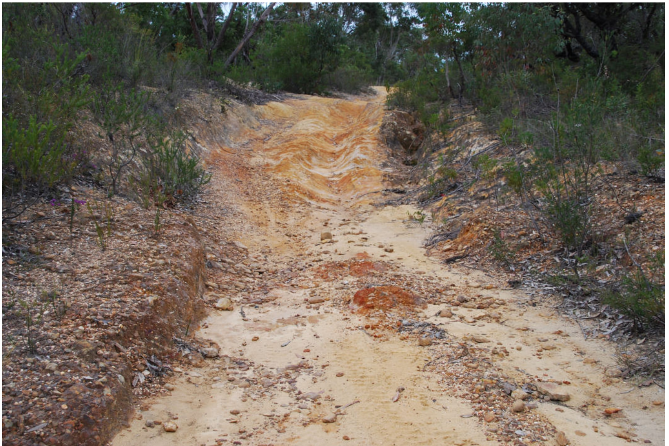
Photo: Road worn through different stone and clay layers
