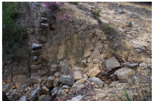
Above: Shows collapsed northern abutment and washed out area behind wall, can see dozed-in fill including timber and shaped stones.
