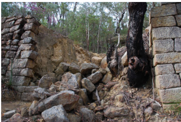
Above: Southern abutment and collapsed northern abutment and filled space between washed out, taken from below base of walling.
