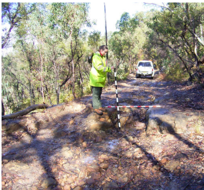
Above: Eric Metzke showing the depth of the washouts in a section of the road which is trafficable.
