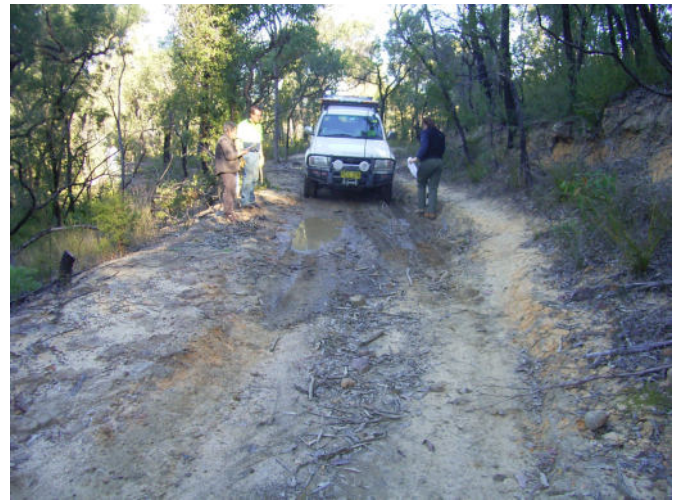
Washout below both sides of road
