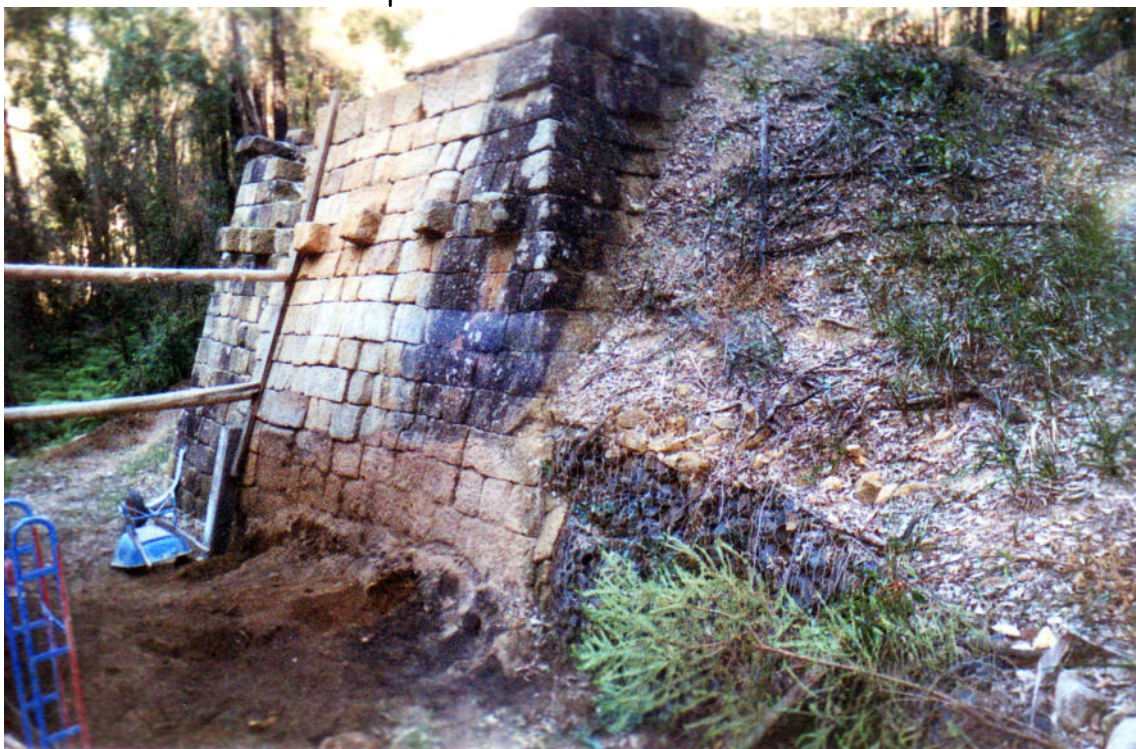
[Southern abutment with decking removed]
