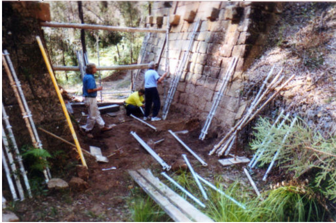
Installing the scaffolding
