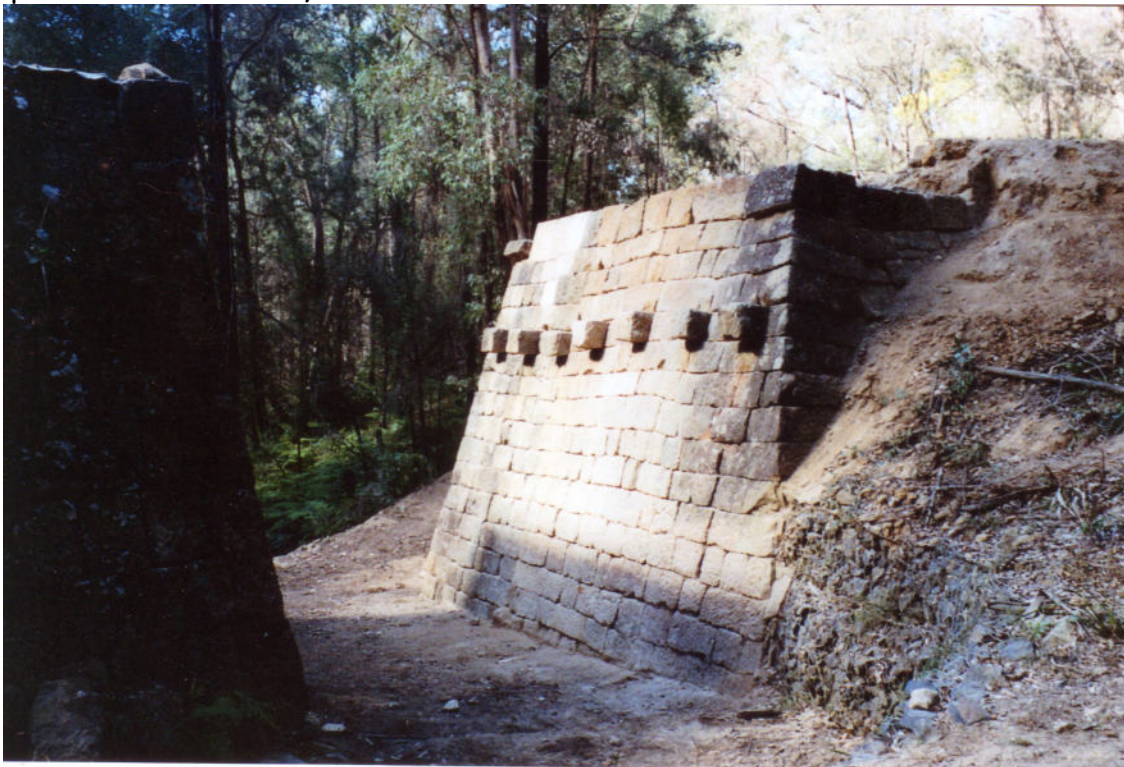
The southern abutment of Clares Bridge restored.
