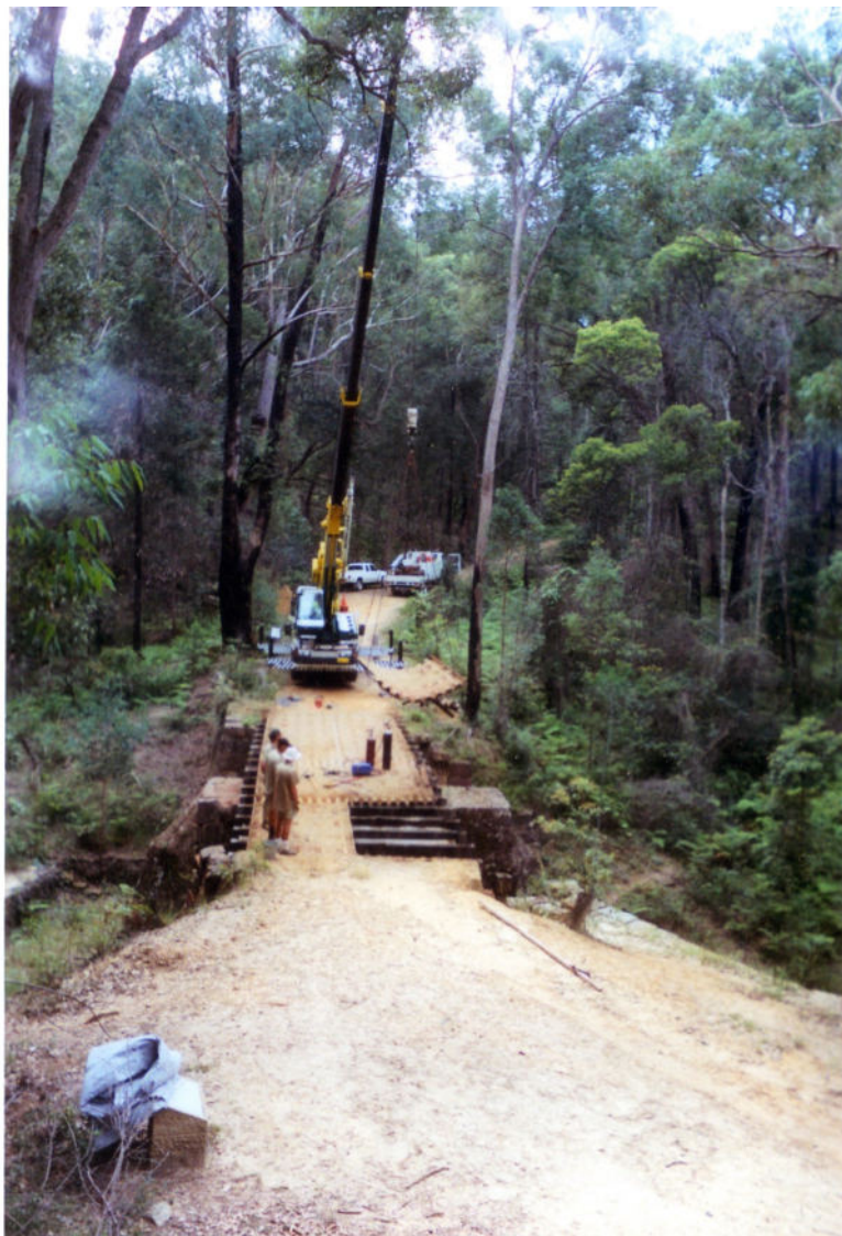
[Demolition of Clares Bridge decking - lifting off the first sheet of metal decking.]
