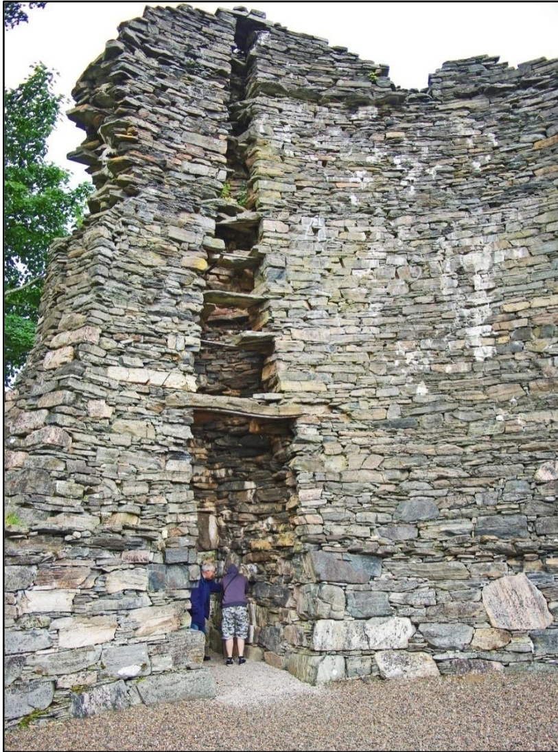
An inside view of Dun Telve, showing the variety of stones used in its construction. The wall is hollow in parts to provide space for the internal staircase.
